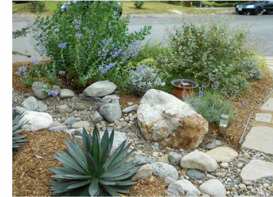
SUSTAINABLE FEATURE: A dry river bed is an area designed to slow heavy flows of water from rainfall and correct erosion problems. It is made up of a shallow swale lined with stone large enough to slow the speed of storm water and prevent erosion.
