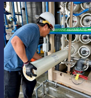
RO Element Installation
