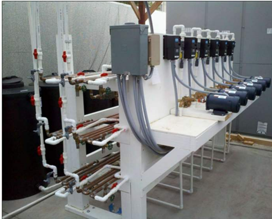
Figure 4-8: Example of Flow-Through Pipe Loop System
